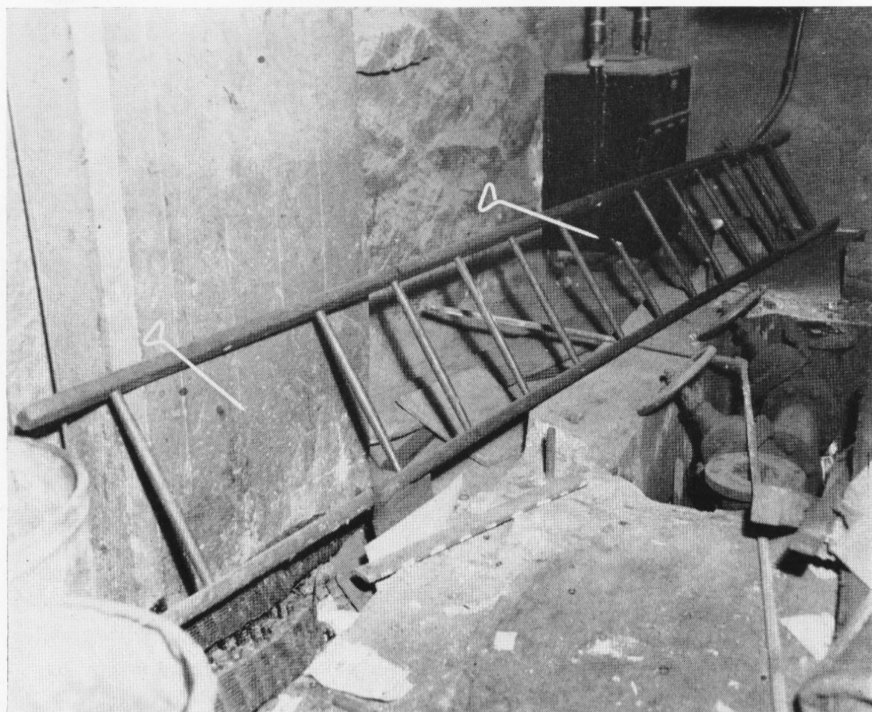
Two missing rungs and a broken one. This ladder is absolutely no good and a man would run quite a risk trying to climb it. With a split side rail the whole structure would topple under a man's weight. Don't take the chance, use a good, safe, steady ladder.
